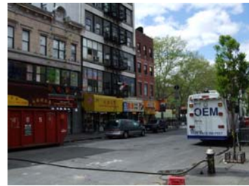
Grand Street fire resulted in 1 fatality and economic impact to over 30 businesses
